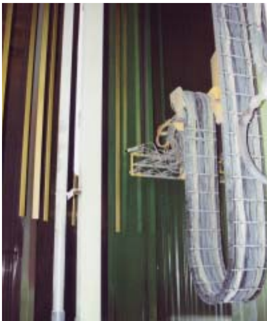
Powder application in a vertical coating system.
