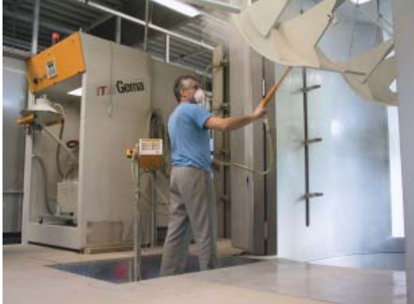
Impressive dimensions: the coating line at the company Haslach was designed for parts measuring up to 2.4 metres wide and 7 metres long.
